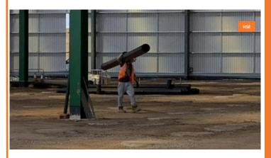
The Health and Safety Executive (HSE) have shared an image of an activity that was observed on a large commercial build. The worker in the image was carrying a large and awkward-tohandle pipe across site, rather than using handling equipment.
