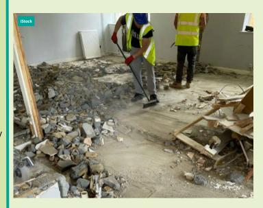
The Health and Safety Executive (HSE) have released an image taken during its Dust Kills Health Campaign on a construction refurbishment site in NW London. The image shows drysweeping taking place indoors without all the necessary dust control measures in place.
