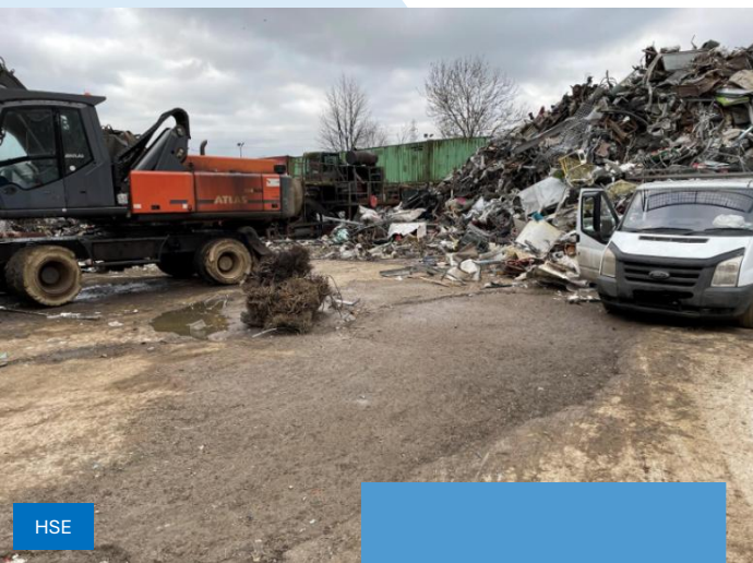
The scrap yard with an unstable metal pile
